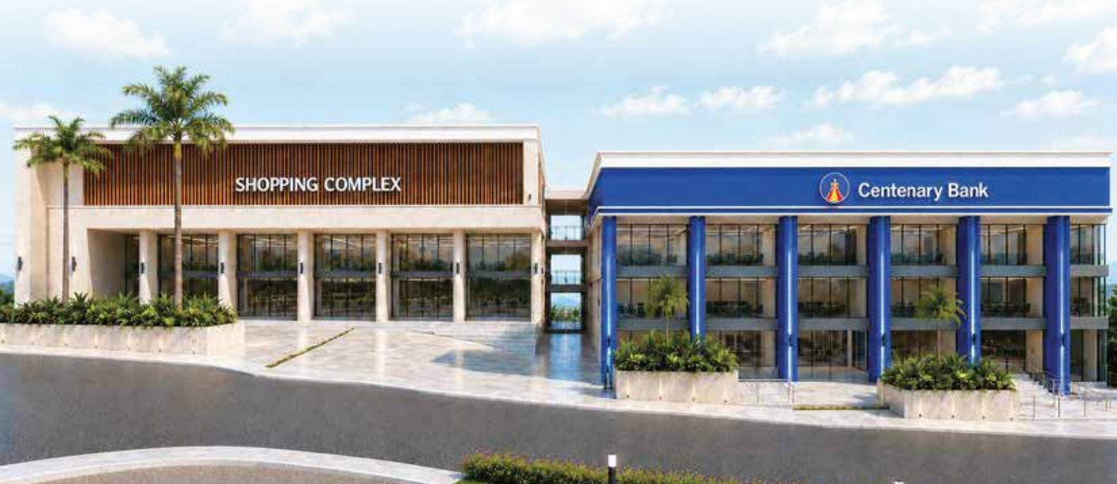
Impression of the AMDEF House, being constructed in Mbarara City, besides the Catholic Social Centre - Uganda Martyrs
